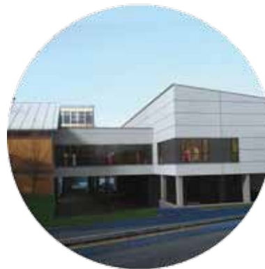
Lagan Valley Hospital Theatres
