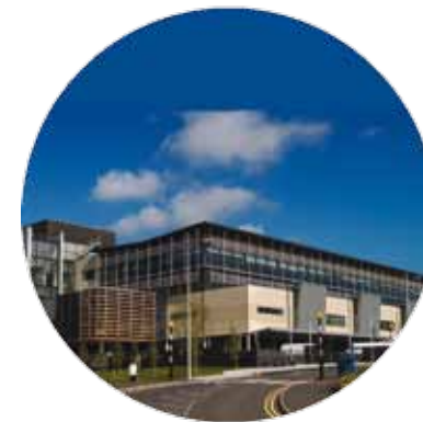
Ulster Hospital Critical Care Block
